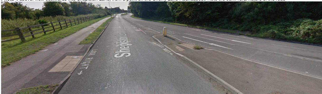
Photo 2 above: existing pedestrian crossing point with tactile paving at the narrow end of the triangular island leading from the Cherry Lane roundabout
