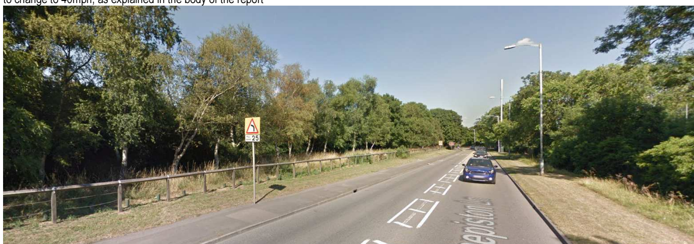
Photo 25 above: looking eastwards with bend warning sign and 'advisory speed' sign, and centre hatching introduced in 2006 (see main report)
