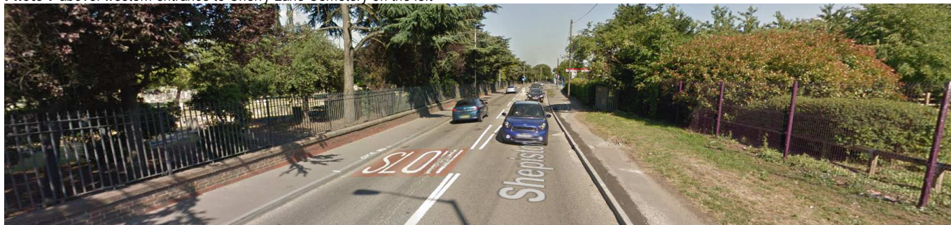
Photo 8 above: Cherry Lane Cemetery wall and railings on left. Note start of centre hatching and 'SLOW' marking with additional red antiskid emphasis
